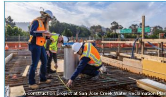
A construction project at San Jose Creek Water Reclamation Plant.
